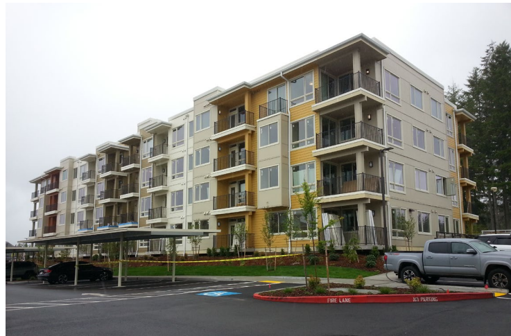
Owner-Build Construction Mid-rise Apartments over parking garage
